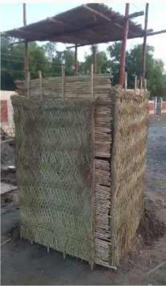
On dated 17th September 2022: SRSO District Khairpur Team installed one straw-made Echo Friendly Pit latrine initially as a pilot basis at Village Sohu Kanasra UC Sohu taluka Kotdij. Financially supported by Waheed Ali & Maria Relief Kitchen.
